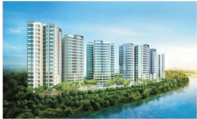
Project Title: The Estuary Contractor: Great Resources M&E Contractor Pte Ltd Fan supplied: Axial, Cabinet & CIL
