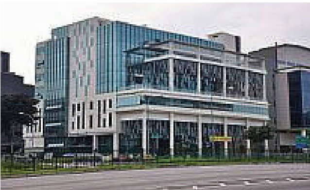
Project Title: Suki Sushi Contractor: Natural Cool Airconditioning & Engineering Pte Ltd Fan supplied: Axial, Cabinet, CIL & Propeller
