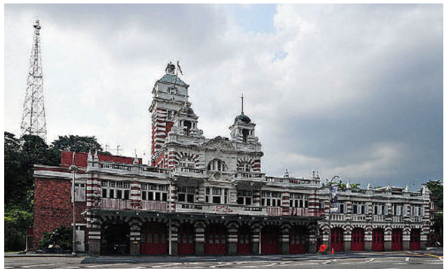
Project Title: Central Fire Station Contractor: BNF Engineering (S) Pte Ltd Fan supplied: CIL & Propeller
